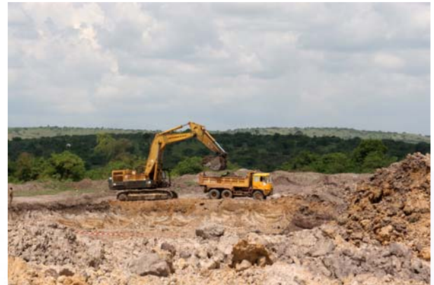
Excavation Solar water pumping Scheme to Kyenjojo Town Council county - Isingiro District
