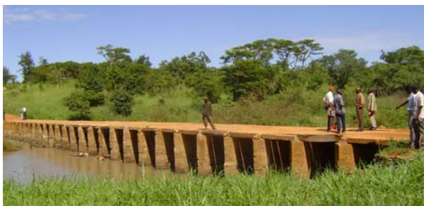
Assessment of Aswa Bridge in Gulu
