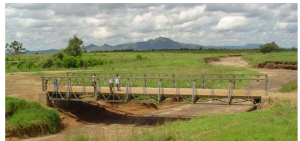
Assessment of Nalakas Bailey Bridge, Kotido
